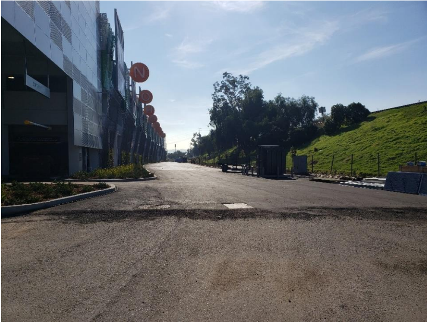
Back of Parking Lot Structure
